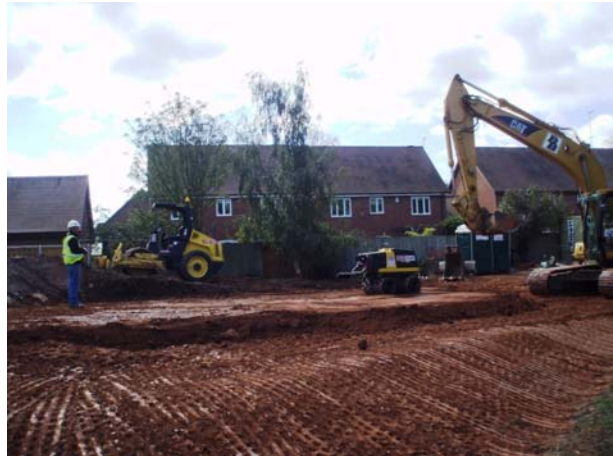
Clay embankment construction and compaction
