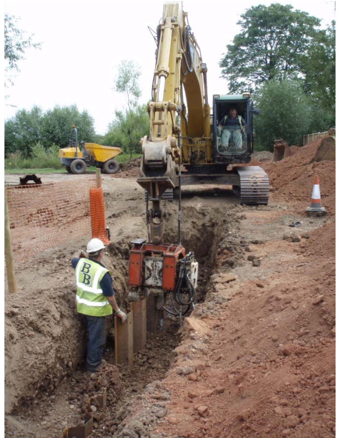
Millers Bank embankment sheet pile cut off
