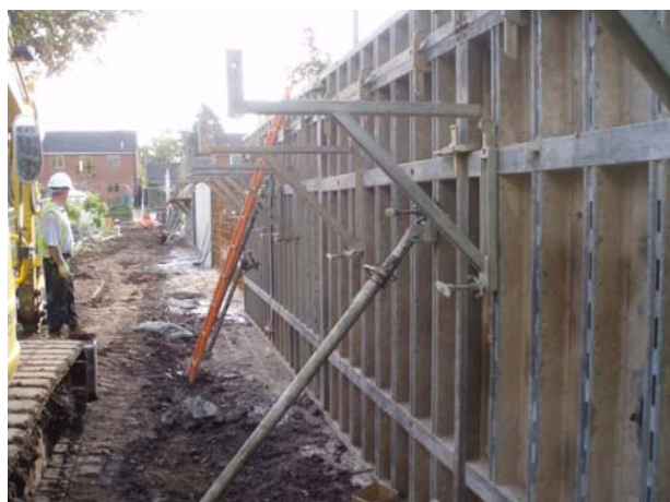
Flood wall construction
