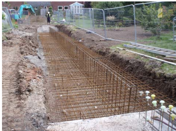
Flood wall foundation construction
