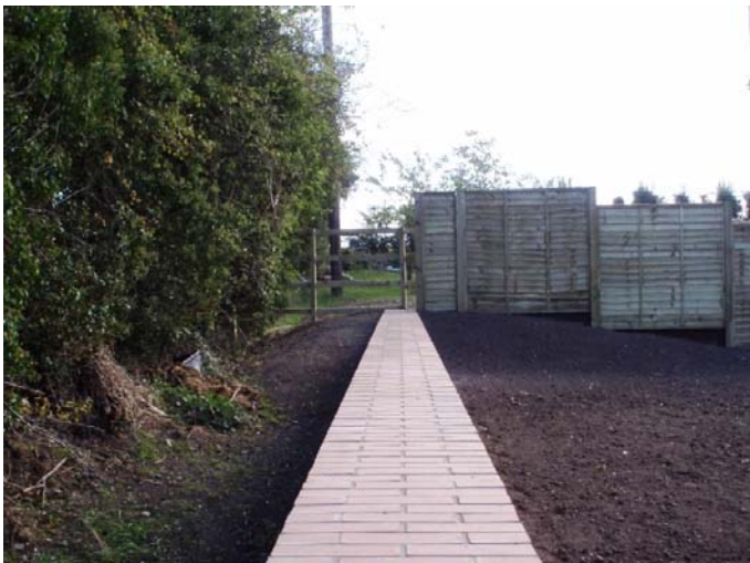
Finished flood wall joining clay core embankment
