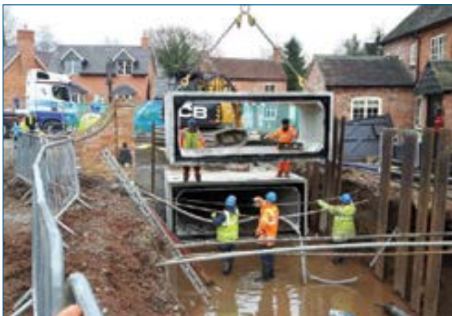
A section of the Snitterfield bypass culvert being installed
